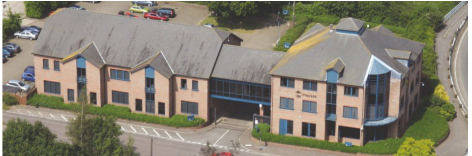
The Plextek Building near Cambridge in the UK
